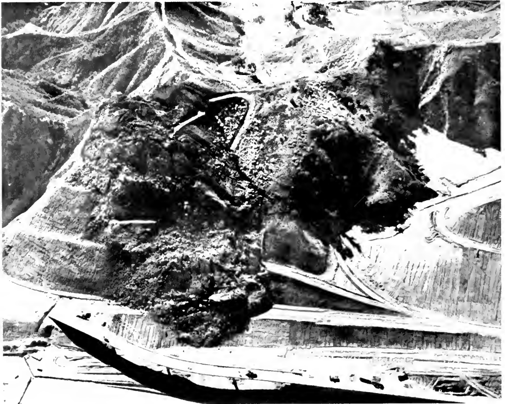
Photo 1. Cut slope failure on Route 5 between route 5/14 and Route 5/210 Interchanges
